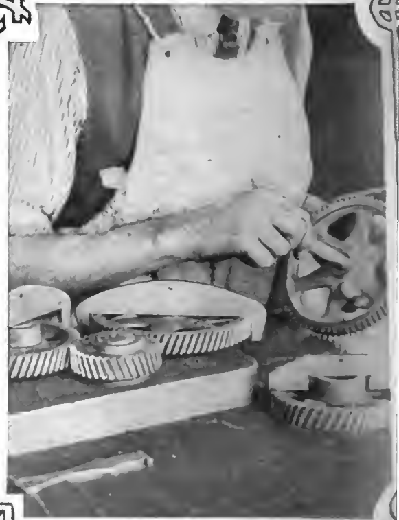
C—Special Form of Equipment Designed to Test Gears for Centers, Bores, and Critical Dimensions
